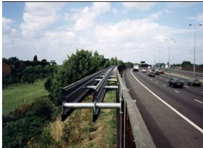
Figure 4.1: Multiple-edged outdoor noise barrier design developed using BEM simulations [16].
